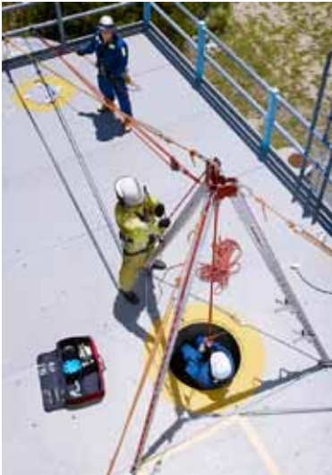
Image: Courtesy of Ferno Simulated confined space access using Arachnipod
